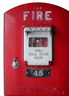
Old Fire Alarm Pull Box
