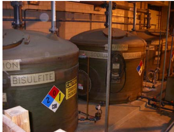
Sodium Bi-sulfite, a de-chlorination chemical Photo Source: Northeast Ohio Regional Sewer District
