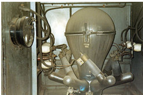
Mercury Arc Rectifier; Photo Source: Wikipedia
